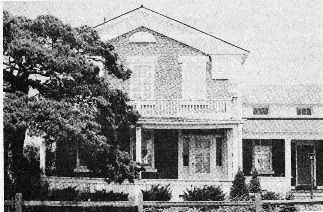
Former F. J. Hill cobblestone on the Ridge in Cambria is a charming example of Late Period workmanship. Walls were veneered with ovate, lakewashed stones; material was cleverly sorted to be practically exacting. Study gable end which faces the road. Stones are of various colors, but grays and browns predominate. But when bathed in full sunlight, walls have an overall sheen. Cobblestones were set vertically in continuous "V" channels without embellishing the vertical joints. Notice Elliptical fan at Gable's Peak with curve of fan enhanced with then stones for artistic sake.
